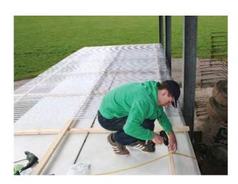
My original idea was using canopies which would have led to adding 3 canopies to the container in total... instead I decided to add a roof construction to the whole container. On top of a simple wooden structure corrugated plastic plates were screwed. The simplest and cheapest solution. At least I thought that at the time. Also more on that later...
